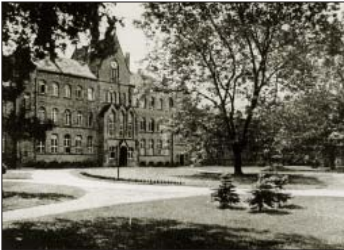
Courtyard of the Hospital and Sanatorium Göttingen (built 1864/1866)
