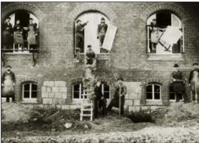
Workmen During the Building of the Hospital and Sanatorium in Lüneburg.
