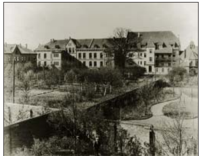
Diverse Buildings of the Hospital and Sanatorium in Wunstorf Womens Houses II and III. Photo from the time of 1925–1927. (Source: Lower Saxony Provincial Hospital Wunstorf.)
