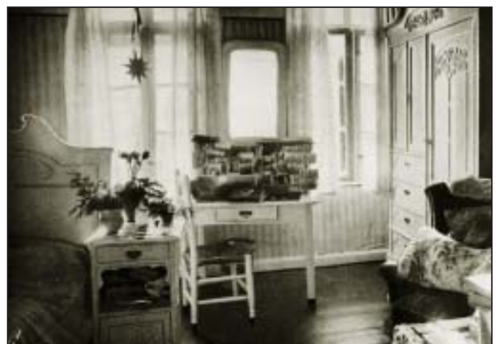
Interior View of a Patient's Room
